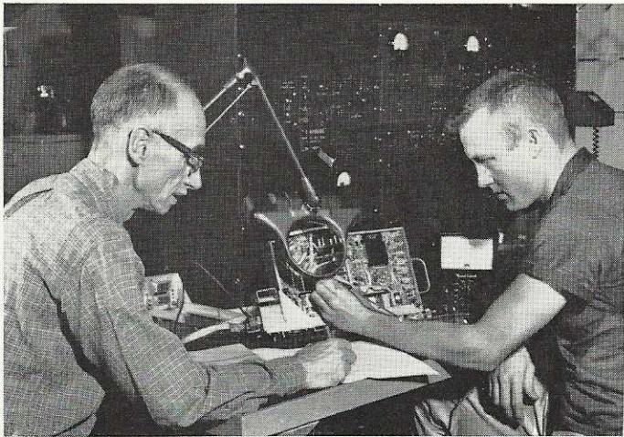
Art Stoner, lead mechanic in the Radio Shop, and Merle Mennenga troubleshoot on a VHF communications receiver, which is used in Frontier's DC-3 equipment.
