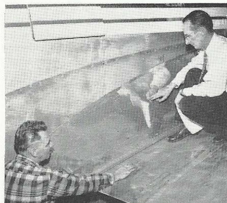
The Challenger 250 kit is being installed on Sunliner 442, which will increase the stability and performance of the aircraft. Assisting in the installation of the wing fillets is Dick Meacham (left) of the Aircraft Conversion Company of Detroit and Fred Elliott, foreman of the maintenance shops. Elliott's hand is on the new wing fillet which is one portion of the kit.
