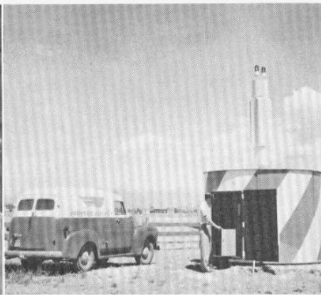
CHECKING . . . Clyde C. Longhart, superintendent of communications checks the automatic radio equipment housed inside the "TVOR" (Terminal Visual Omni Range) located near the Durango airport. This new navigational device "homes in" all approaching aircraft during approaches and let-downs at Durango.
