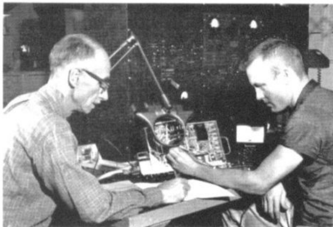
Art Stoner, lead mechanic in the Radio Shop, and Merle Mennenga trouble-shoot on a VHF communications receiver, which is used in Frontier's DC-3 equipment.
