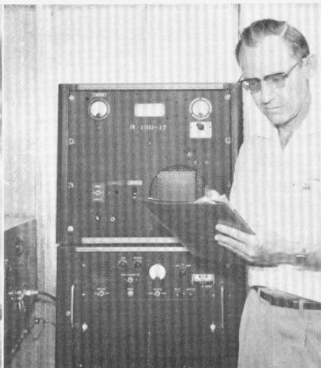
"H" MARKER . . . This provides navigational guidance to aircraft en route between Cortez and Grand Junction, and also aids flights approaching Cortez for a landing. Here again Clyde Longhart makes a check of the equipment at Cortez.
