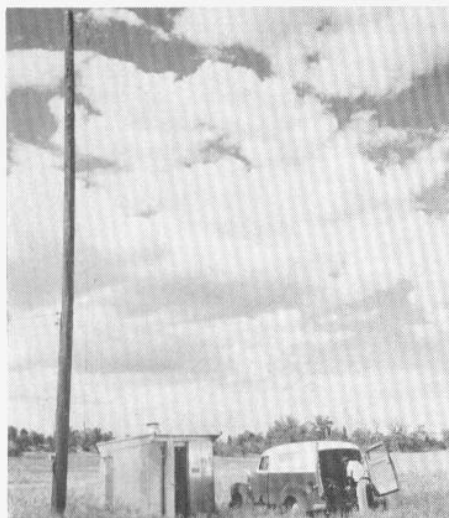
"H" MARKER . . . This provides navigational guidance to aircraft en route between Cortez and Grand Junction, and also aids flights approaching Cortez for a landing. Here again Clyde Longhart makes a check of the equipment at Cortez.
