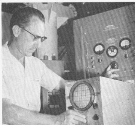
CHECKING . . . Clyde C. Longhart, superintendent of communications checks the automatic radio equipment housed inside the "TVOR" (Terminal Visual Omni Range) located near the Durango airport. This new navigational device "homes in" all approaching aircraft during approaches and let-downs at Durango.
