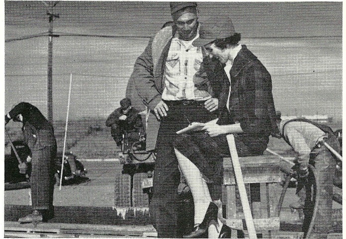
W. K. "Andy" Anderson, superintendent of construction on Frontier's new office building, dictates his New Year's resolution to do a speedy and efficient job to "Building Progress Girl" Betty Moore. At the time of this picture, the cement airways were being poured in the building's foundation. Betty, by the way, became Mrs. William Moore III, on New Year's Eve!
