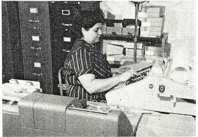
All of Frontier's accounts payable are posted on this Burroughs Sensimatic posting machine. This information is relayed electrically to the IBM key punch in the foreground which turns out punched cards used in preparing Frontier's checks, vouchers, monthly ledgers, and to check bank reconciliation. Elmergene Yantorno operates the bank of accounting machines.
