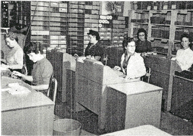
The many thousands of IBM tabulating punched cards which are handled by Frontier's IBM Department are first processed by the girls in the key punch and card verifier section. Each card can be punched with up to 80 columns of information. Left to right are (row 1) Mary Marr, Debbie Moses, (row 2) Elmergene Yantorno, Floy Hildenbrand, (row 3) Alice Solf and Brone Roberts.
